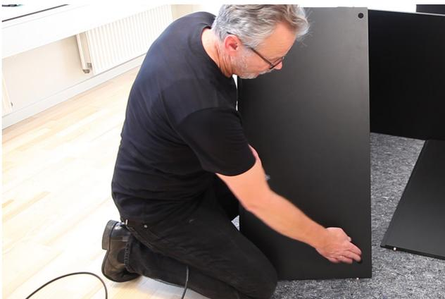
Insert the second Back-Wall part, while making sure the overlaps match, and both parts are aligned.
